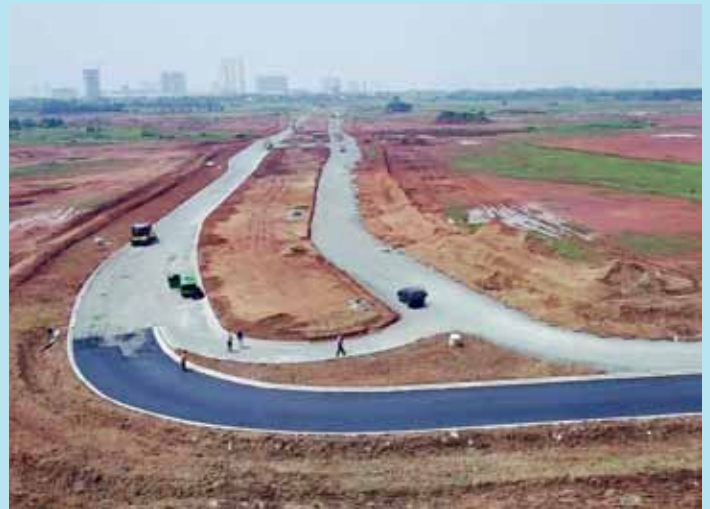
Plastic asphalt-paved roads project by Sinar Mas Land & Chandra Asri in BSD City area.
